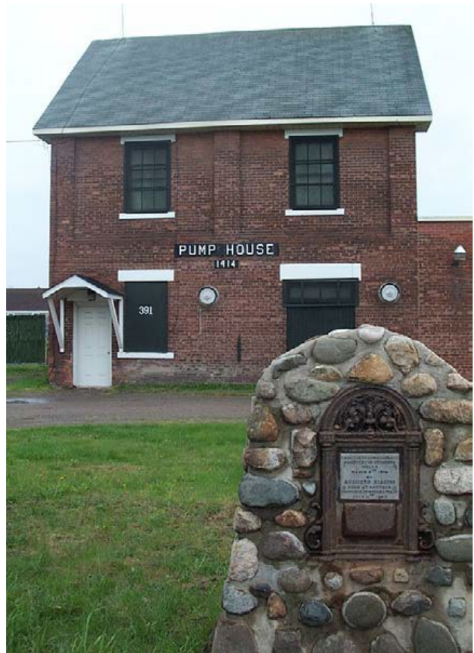
Steelton Pump House established 1914.
