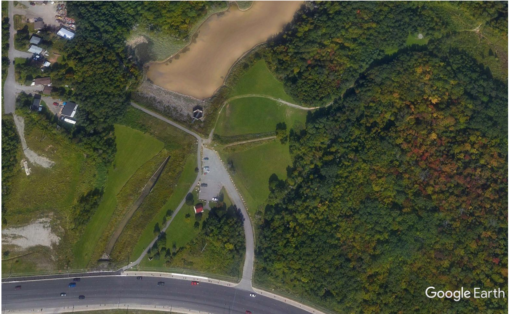
Figure 2: Fort Creek Dam and Reservoir (Aerial view).
