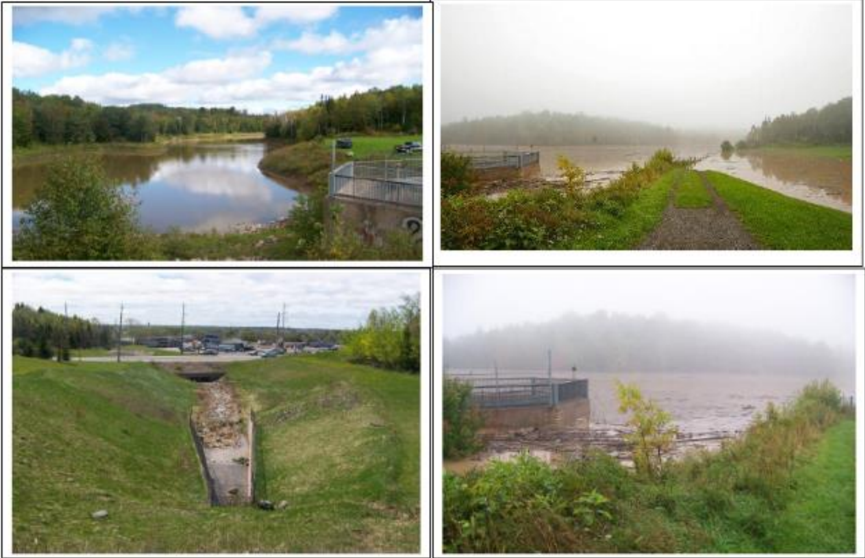
Figure 3: Fort Creek Dam and Reservoir (Dam holding flood flows in 2013).
